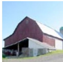
Gambrel Roof (barn) with Shed in foreground
